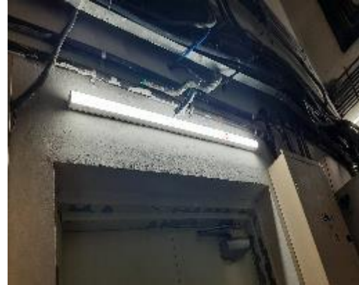
20W LED Tube Fixture
