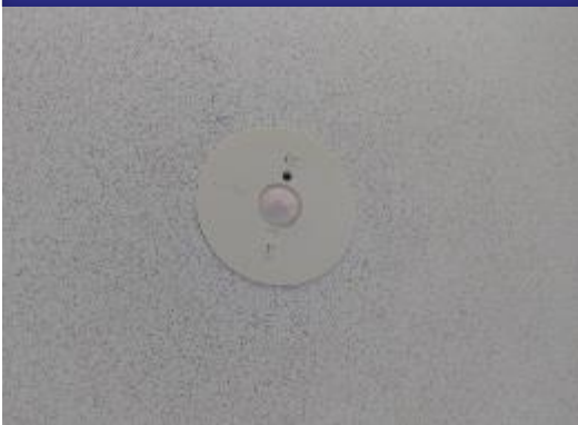
Motion Control Sensor for washroom Lighting
