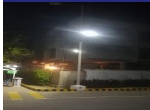
Peripheral light retrofit (250W MHL to 100W LED)
