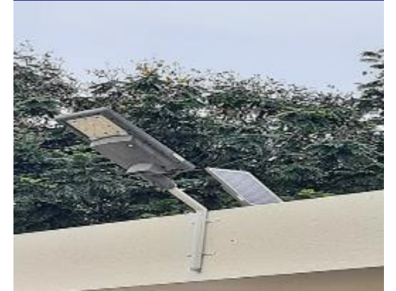
Solar Light Retrofit (250W - 30W)
